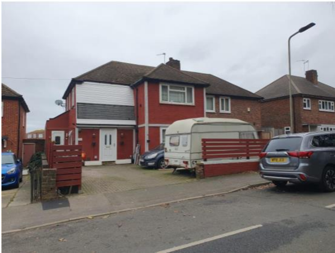
Figure 6: Photograph of the site from the front:
